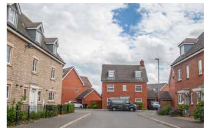
Residential development in Calverton
