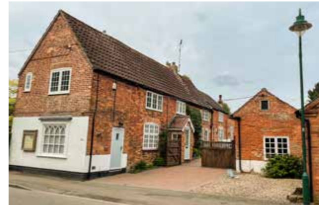
Dwellings with gable ends facing Main Street in Calverton
